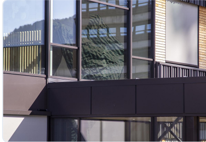
Project B exterior
